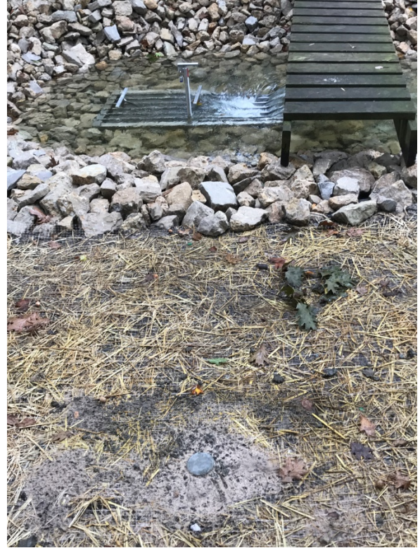
Surveyor benchmark at 869.61' located 13' NW of center of weir opening
