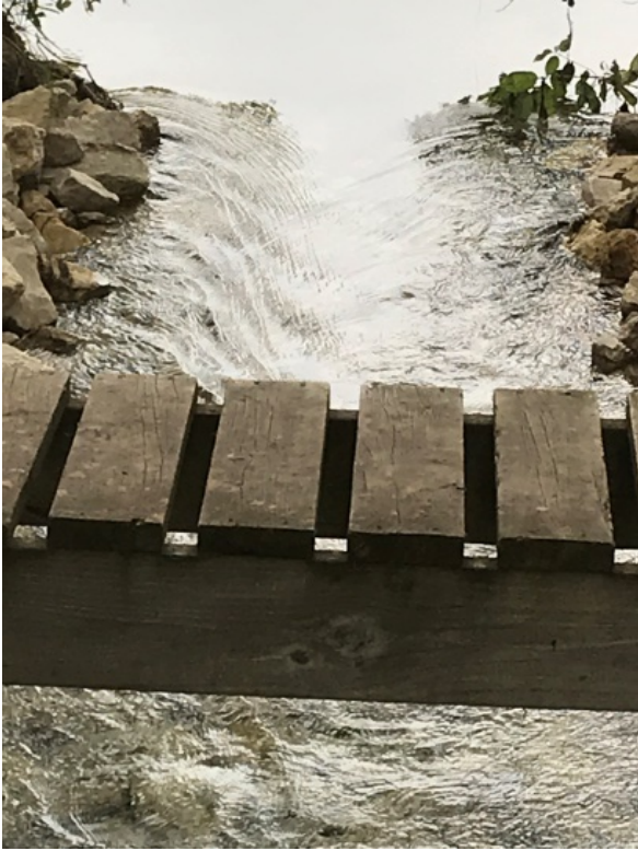
Inlet channel from Lake Irogami. Weir flowing at ~5cfs
