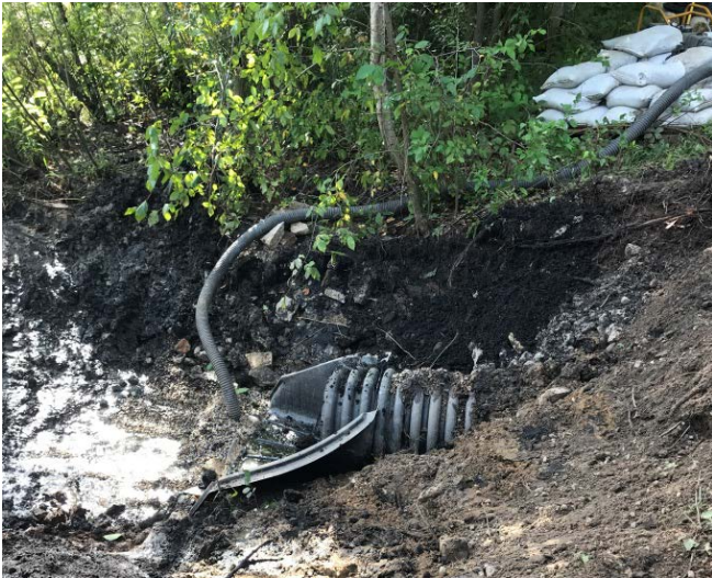
Exit pipe spillway. Infiltrated water pumped to marsh.
