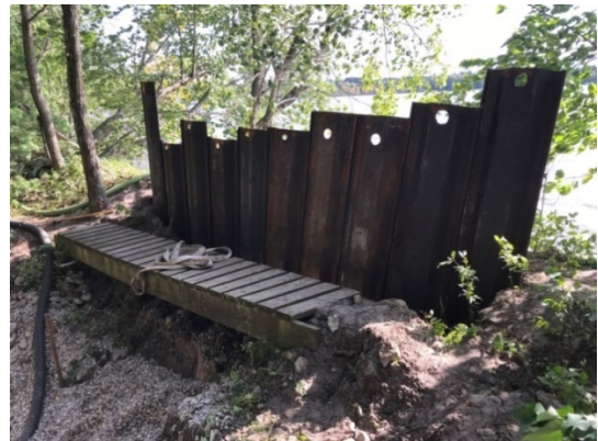
Sheet piling to isolate weir construction area.
