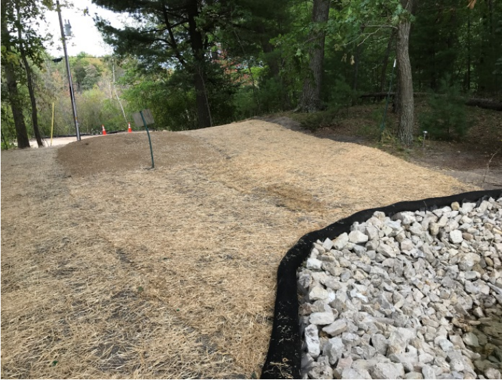
Landscaping at east end of weir. Facing north.
