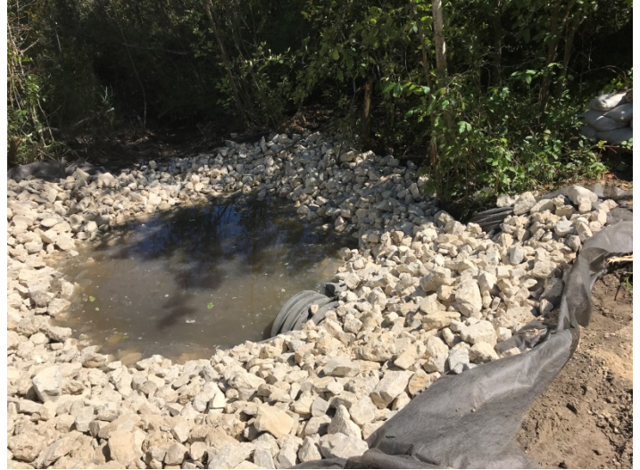
Outlet with riprap and silt barrier installed. (weir not flowing)
