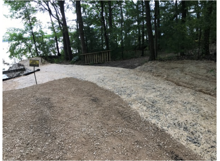
Landscaping at west end of weir. Facing south.
