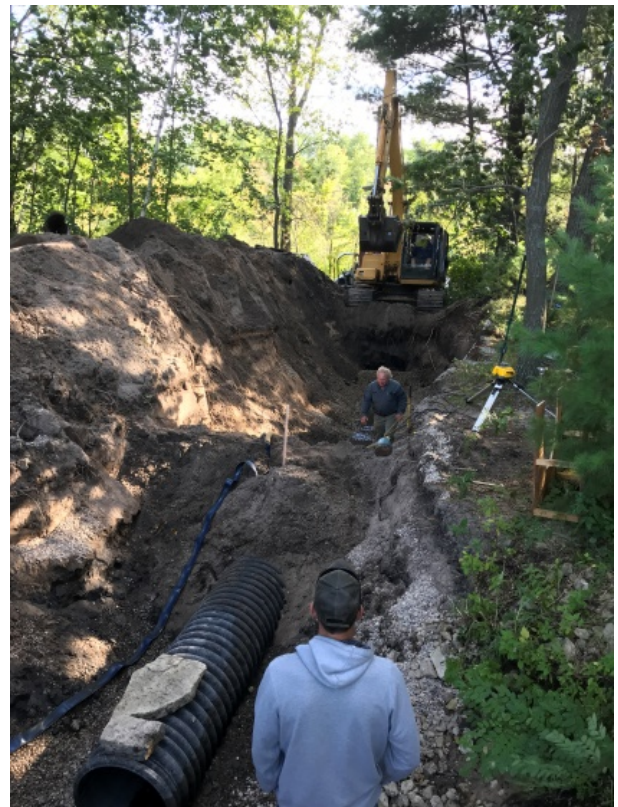
Middle pipe section installed first. Gravel placed under discharge pipe.
