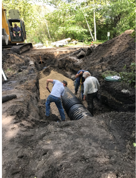
Discharge pipe elevation set and stabilized with gravel.
