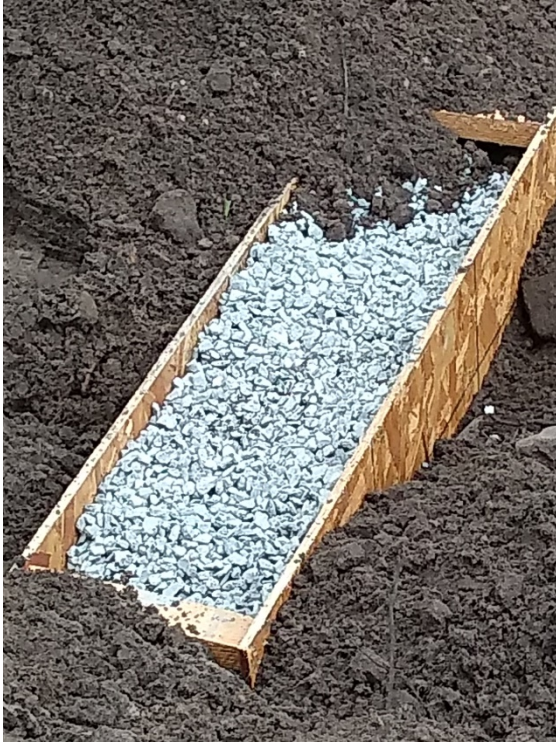
Bentonite saddles used to stabilize discharge pipe.
